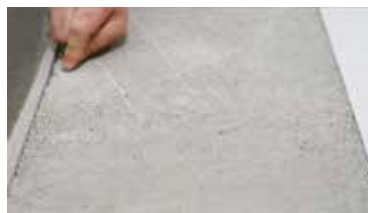
CEMENT-BASED SCREED checking hardness and cleanliness
