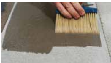
CONCRETE checking absorption
